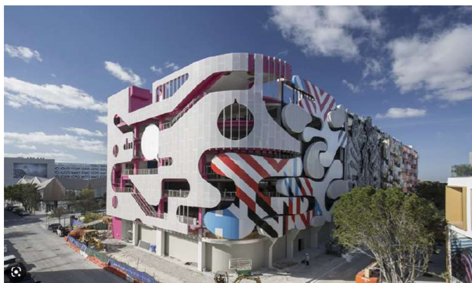
Source: http://modernmag.com/miamis-design-district-gets-a-surrealist-inspired-parking-garage/ Museum Garage for Miami Design District. Photo by Robin Hill
